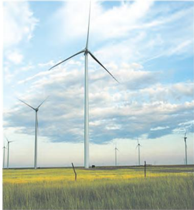
Spearville 2 Wind Energy Facility in Western Kansas
